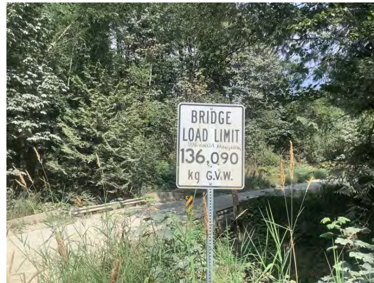
Load Rating Sign
