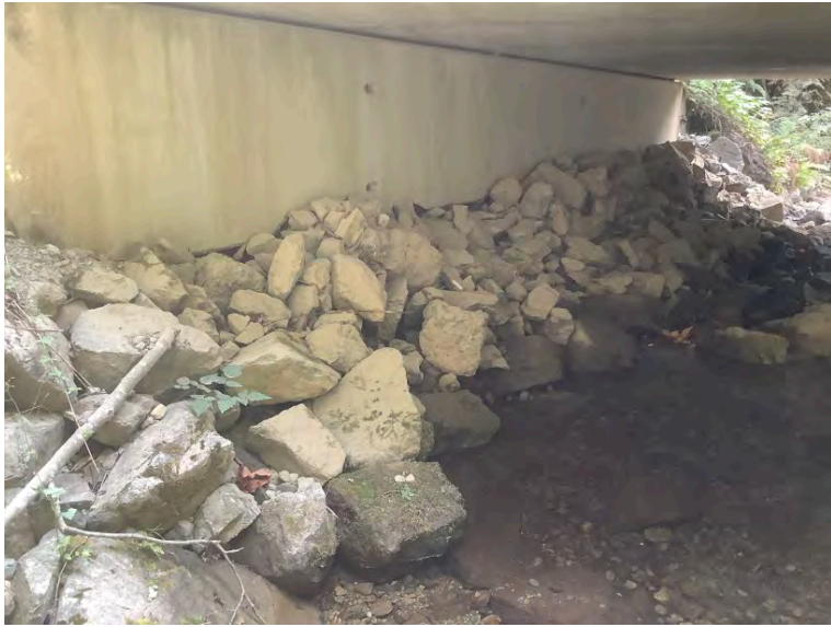
Left Bank Abutment when facing downstream
