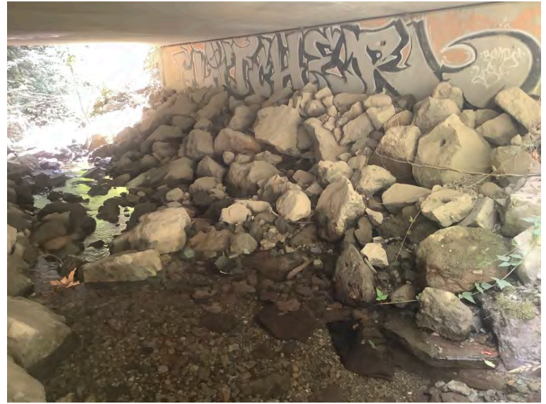
Right Bank Abutment when facing downstream
